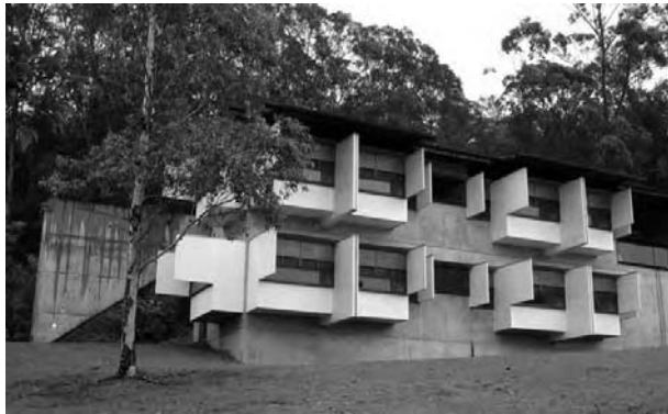
Figure 16 Windows at Glenn Murcutt's Boyd Education Centre in New South Wales, Australia, showing layering of façade elements, including fins, overhangs, and operable shading devices
