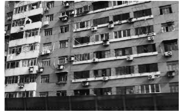
Figure 5 Many residents install their own air conditioners
