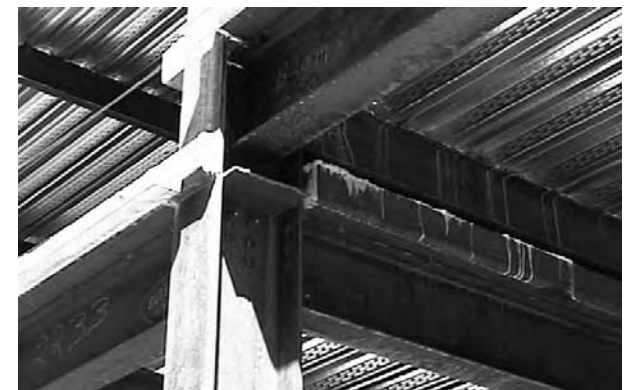
Figures 7 and 8 Structural steel construction
