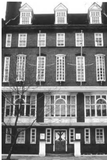
Figure 14 Old Swan House, London, U.K. by Norman Shaw, 1876 (example of maritime architectural form)
