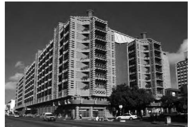
Figure 8 Shading can be incorporated into mid-rise and high-rise buildings. This office building in Harare, Zimbabwe, uses shading to reduce heat gains and heavy construction to moderate indoor temperature swings. Ventilation is provided by fans, but there are no chillers.
