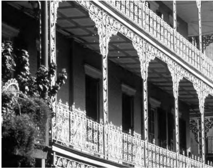
Figure 12 Porch and balconies as buffer zone to housing, New Orleans, U.S. (example of subtropical architectural form)
