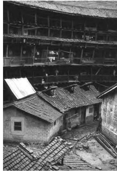
Figure 13 Inside circular housing, Fujian, China (example of subtropical architectural form)
