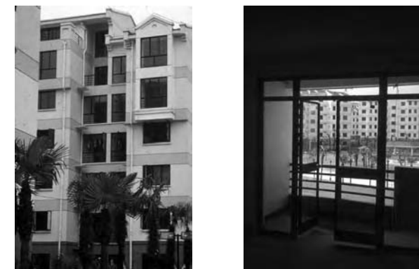
Figure 2 Daylighting in a multifamily residential building in the Pudong region of Shanghai
