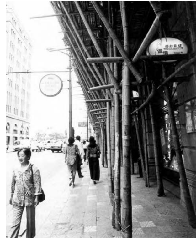
Figure 1 Use of renewable resources in construction, such as bamboo scaffolding on this Shanghai construction project
