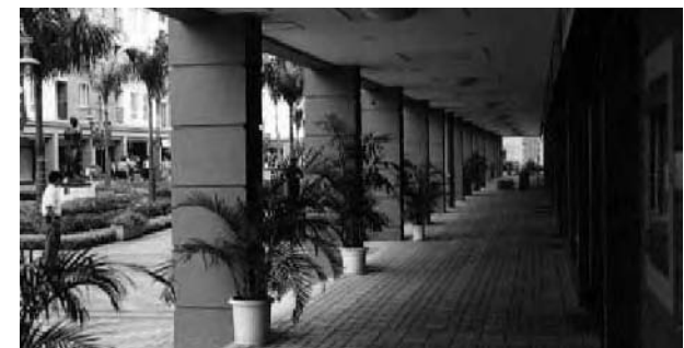
Figure 4 Covered outdoor walkways provide shaded areas
