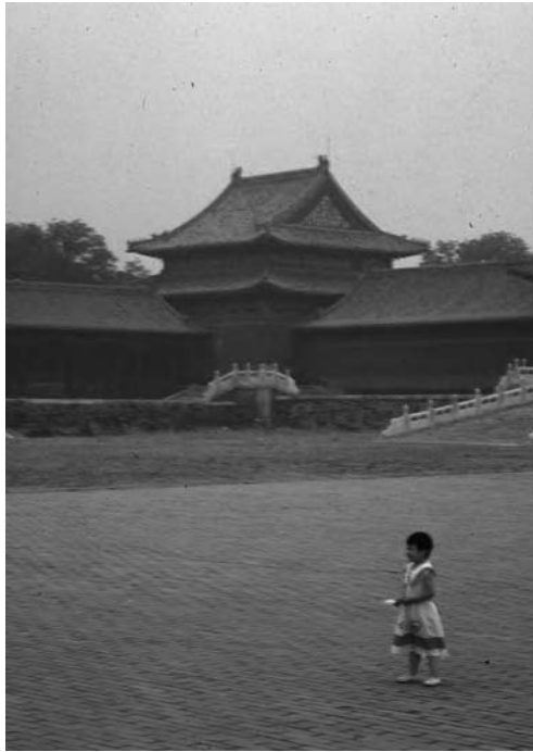
Figure 3 Overhanging roofs on buildings in the Imperial Palace in Beijing protect indoor spaces from direct sunlight in summer
