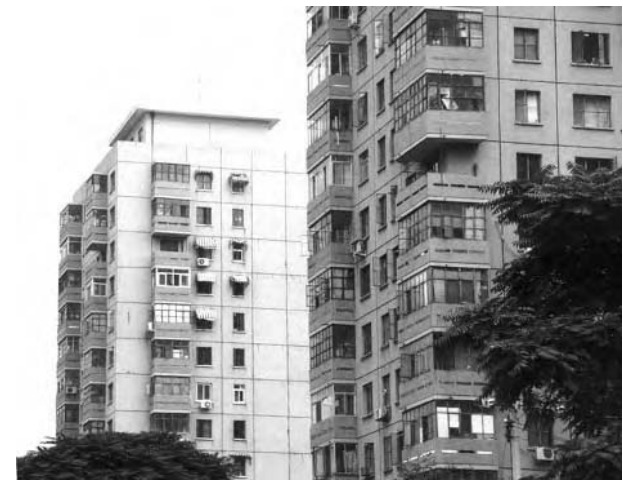
Figure 6 Permanently closed-in balconies create a greenhouse space that substantially increases air-conditioning requirements
