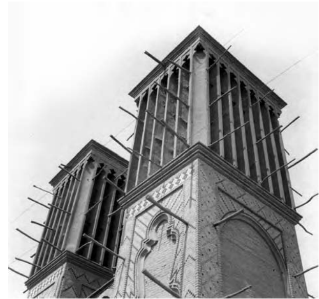
Figure 6 Traditional ventilation technology: wind towers
