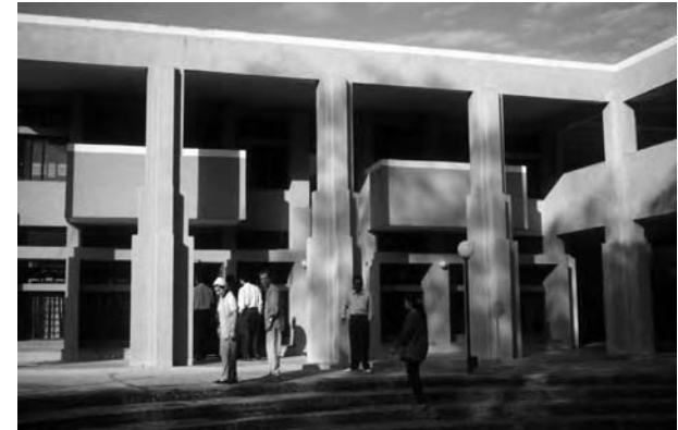
Figure 7 Shading is used successfully in this school near Ahmedabad, India
