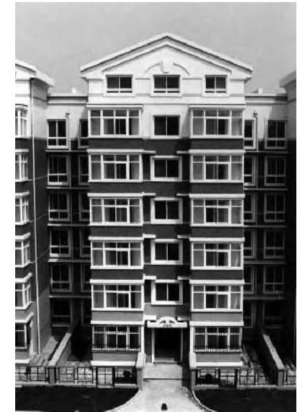
Figure 2 Typical six-story building construction at Hui Long Guan development
