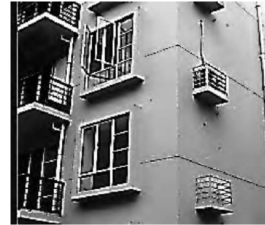
Figure 40 Existing overhangs and air-conditioner units at Shenzhen Wonderland
