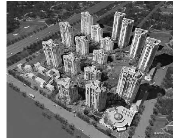
Figure 2 Vanke's original design for Beijing Star Garden master plan (north is to the upper right)
