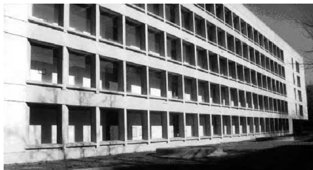
Figure 10 This MIT building uses inset windows to create deep overhangs and fins
