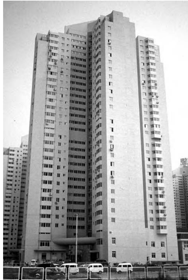
Figure 6 Which way is south? This high-rise residential building in Beijing lacks any reasonable relationship to the sun.
